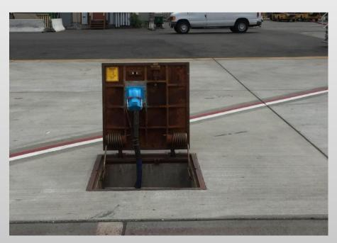
Safety concerns were raised after the existing 400 Hz power stations were installed.
